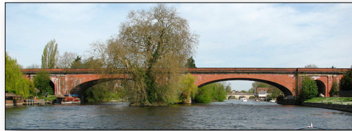
Maidenhead Railroad Bridge, England, I. K. Brunel, 1838.
