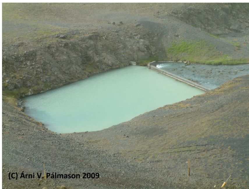
Figure 15. The leak from the Sigalda dam captured and measured
